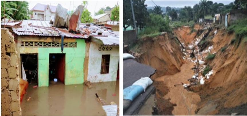
Fig. 14. Erosion and Inundation at Kinshasa
